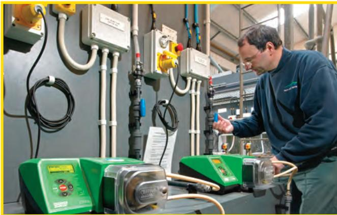
500 series pumps replaced troublesome diaphragm pumps for coagulant dosing
