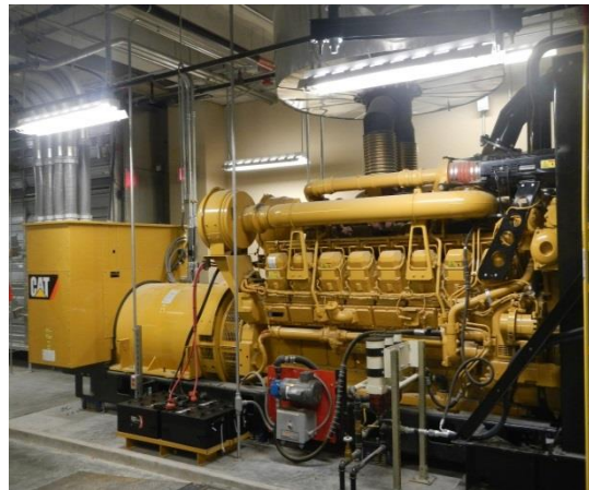
Back-up Generators / UPS System (Uninterruptible Power Supply)
