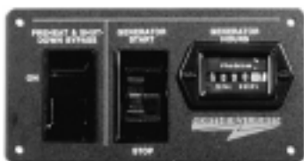
S-1B control panel
