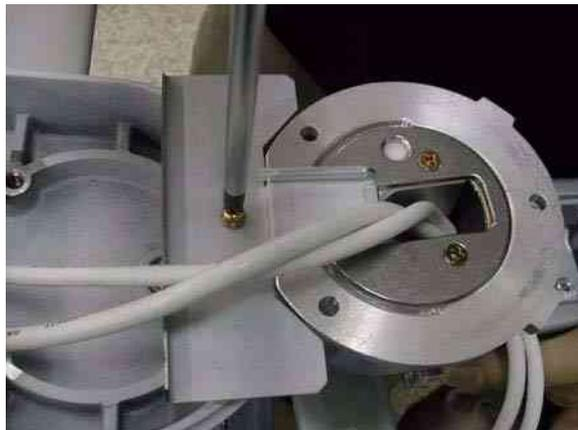
Figure 8-40 Installing OP Bracket
