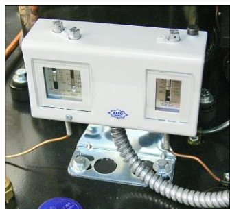
Figure 4-3 Refrigerant Pressure Control (Dual model shown)
