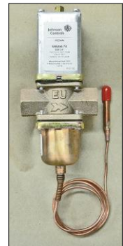
Figure 2-2 Automatic Water Regulating Valve
