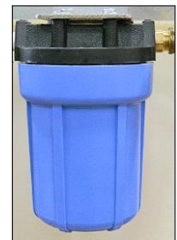
Figure 5-2 Supply Line Filter
